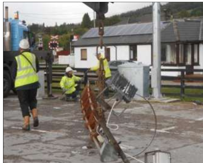
Removal of old lighting towers at Corpach Basin
