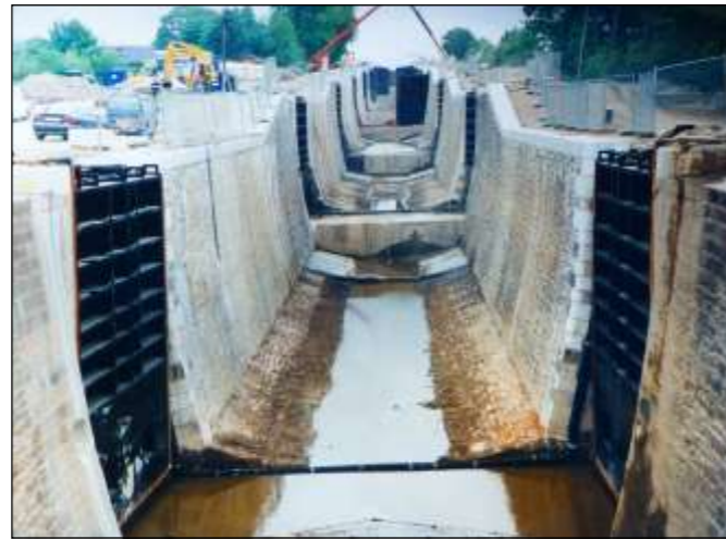
The structure of Neptune's Staircase exposed to view during repairs. Photo: Alex Gillespie, courtesy of Scottish Canals
