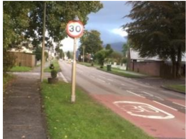
Sign on entry to 30mph area travelling from the West. No countdown chevrons. Poor road markings.
