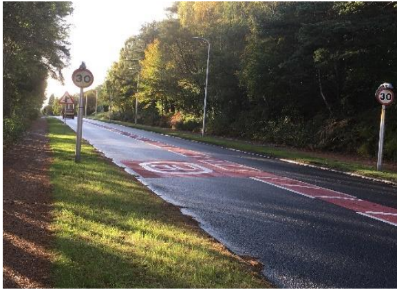
Signage on entry to 30mph area from Banavie bridge. No countdown chevrons from 40mph area. No safety camera van signs. No welcome village signs.
