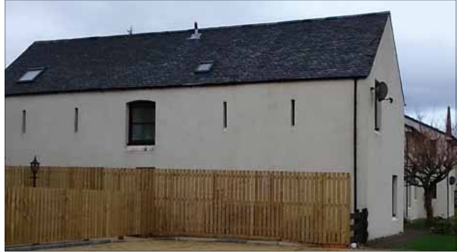
The Kilmallie glebe barn, now converted to residential use, but still a lovely example of the uniquely characteristic Lochaber barns - they were often built into a hillside, known then as a 'bank barn'.
