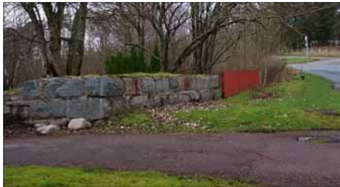
The remains of one of the abutments of the old bridge that carried the Banavie Branch Railway over the original Blar road
